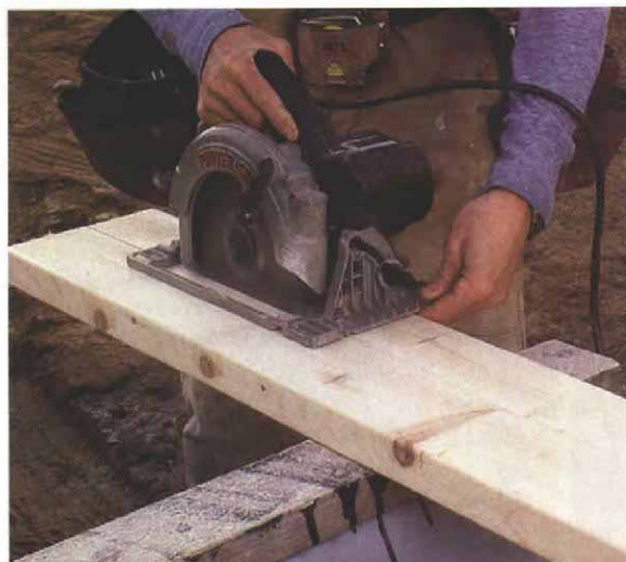
A finger becomes a rip guide in a pinch.
