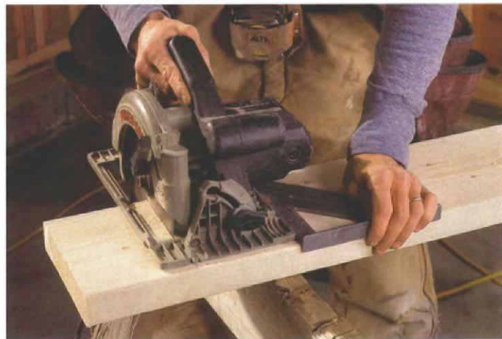
Register the saw against the square to guide the cut.
