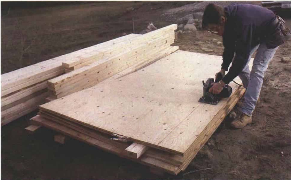
Clamping pliers hold sheet goods together for gang-cutting.
